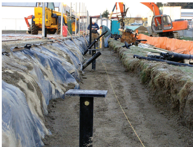
FIGURE 3-3 : New Construction Bracket
