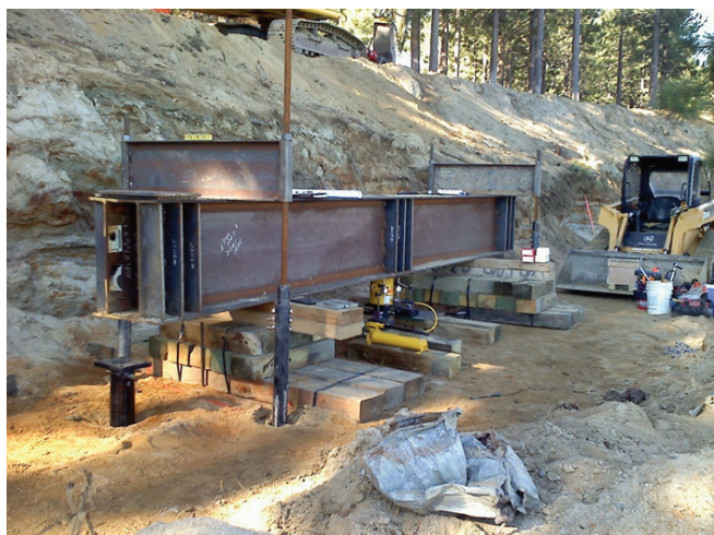
FIGURE 3-16 : Pile Load Compression Test Setup
