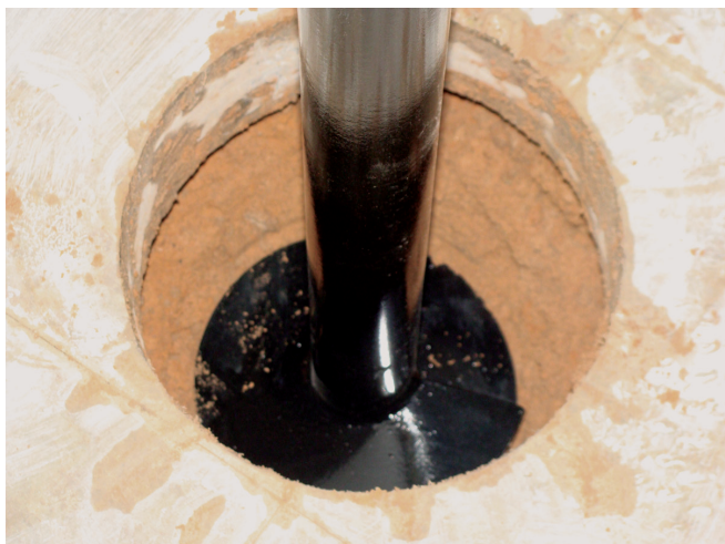
FIGURE 3-27 : Helical Installation Through Concrete Floor Slab
