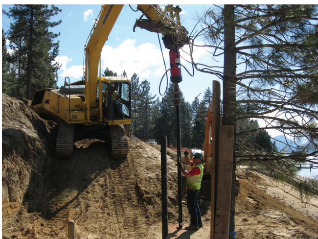
FIGURE 3-24 : Track Hoe Used To Install 5.625" Helical Piles
