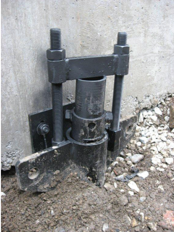
FIGURE 5-7 : Installed Driven Pile with Support Strap Assembly
