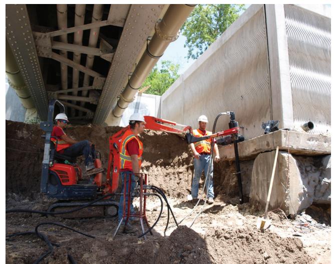
(b) Mini-Excavator Used for Installation
