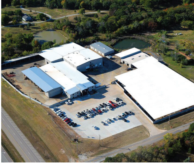
FIGURE 1-2 : Ram Jack Headquarters
