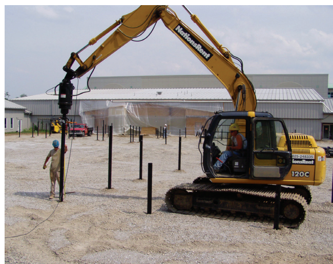
FIGURE 3-25 : Installation of New Construction Piles
