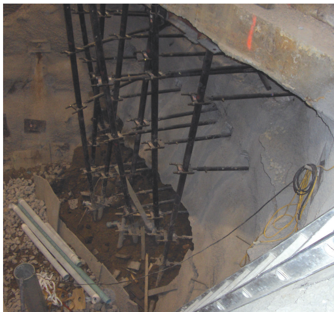
FIGURE 4-6 : Lateral Bracing – (a) Helical Tiebacks and (b) Diagonal Bracing
