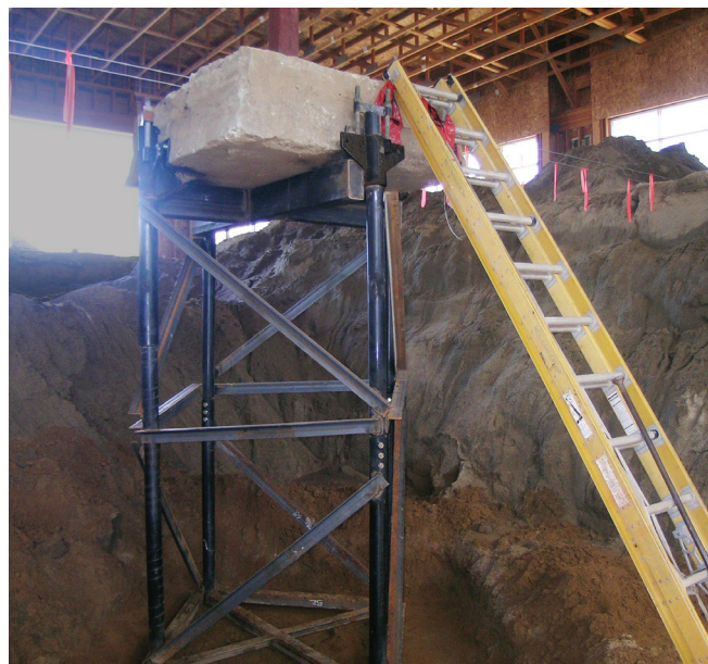
FIGURE 4-6 : Lateral Bracing – (a) Helical Tiebacks and (b) Diagonal Bracing
