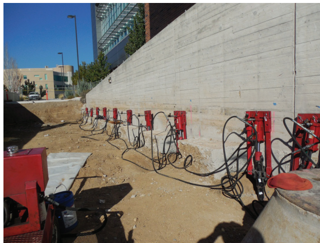
FIGURE 5-9 : Ram Jack Multi-Lift System
